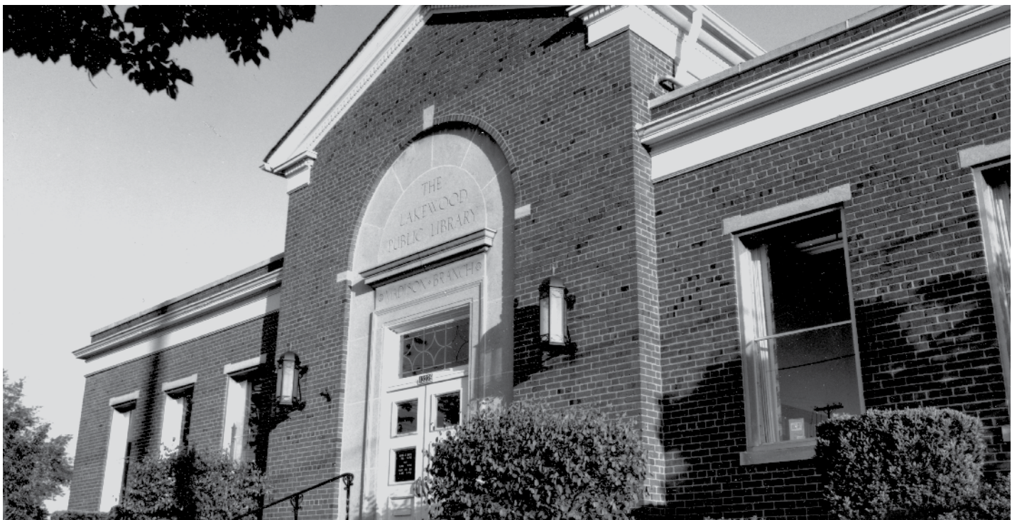
Lakewood Public Library Madison Branch exterior.
